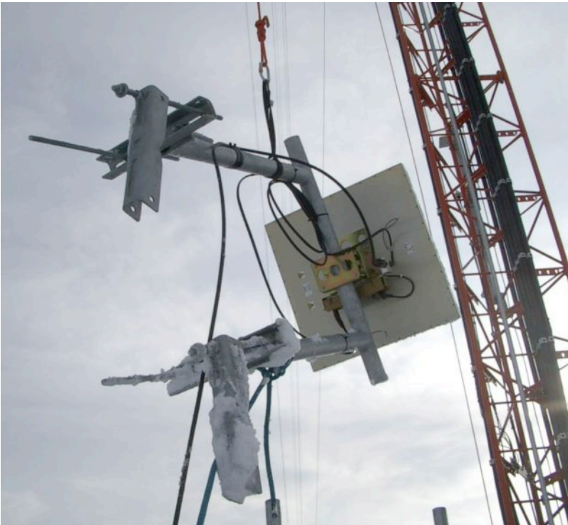
Figure 7.1: An antenna with a standoff bracket being lifted onto a tower.
